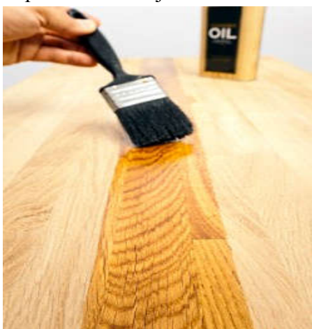
Slika 10 – Prikaz nanošenja ulja kistom ( http://www.house-painting-info.com/wp-content/uploads/2014/06/artimg_applyin_g-tung-oil-wood-countertop.jpg )
