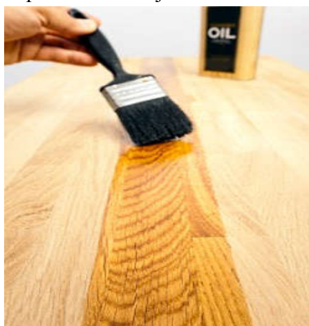
Slika 10 – Prikaz nanošenja ulja kistom ( http://www.house-painting-info.com/wp-content/uploads/2014/06/artimg_applyin_g-tung-oil-wood-countertop.jpg )
