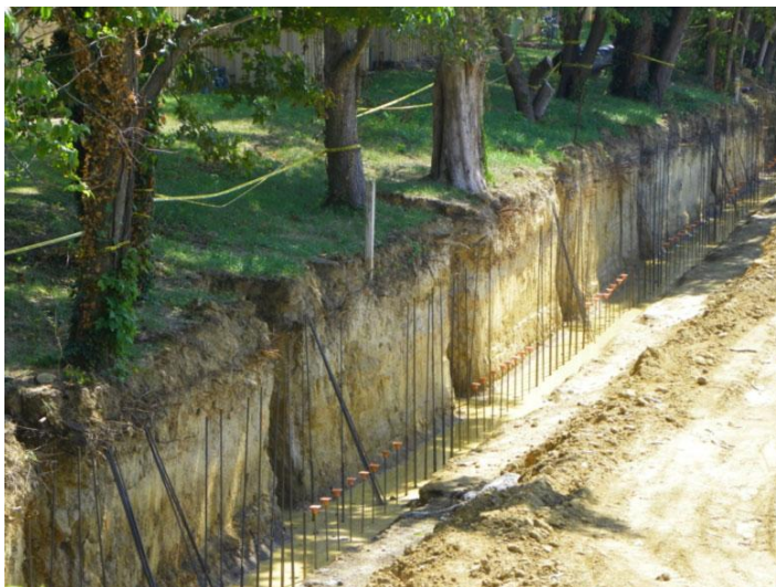
Slika 1. Rov iskopan tijekom građevinskih radova u neposrednoj blizini starijih urbanih stabala. (Izvor: Full circle tree & shrub L.L.C., Construction damage: How to Preserve Your Landscape https://fullcircletreeandshrub.com/blog/construction-damage-how-to-preserve-your-landscape/ (Pristupljeno: 18.9.2021.)
