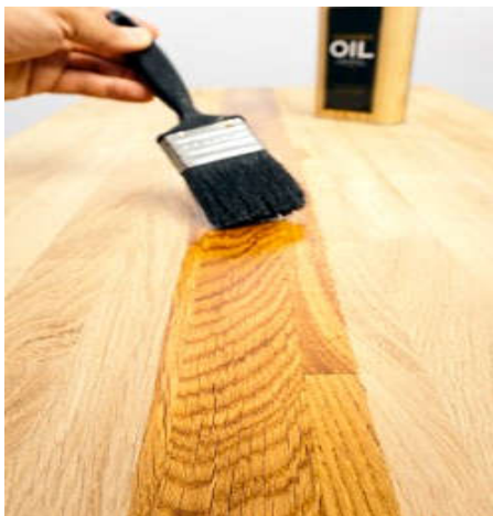
Slika 10 – Prikaz nanošenja ulja kistom ( http://www.house-painting-info.com/wp-content/uploads/2014/06/artimg_applying-tung-oil-wood-countertop.jpg )
